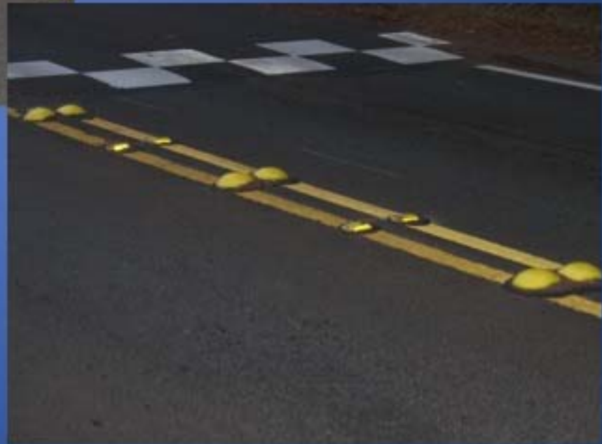
Raised pavement markers to deter crossing of centerline
