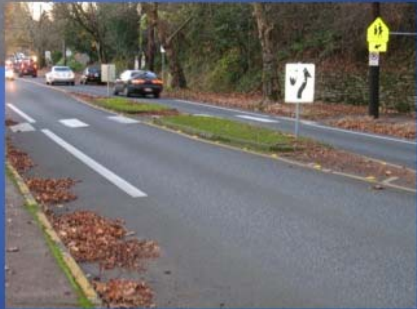
Existing Pedestrian Refuge Island
